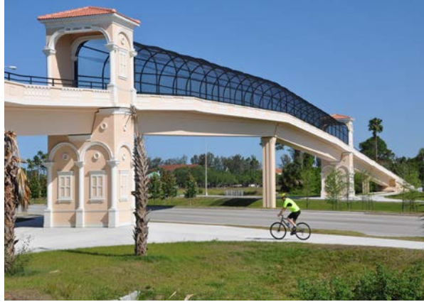
LEGACY TRAIL BRIDGE
